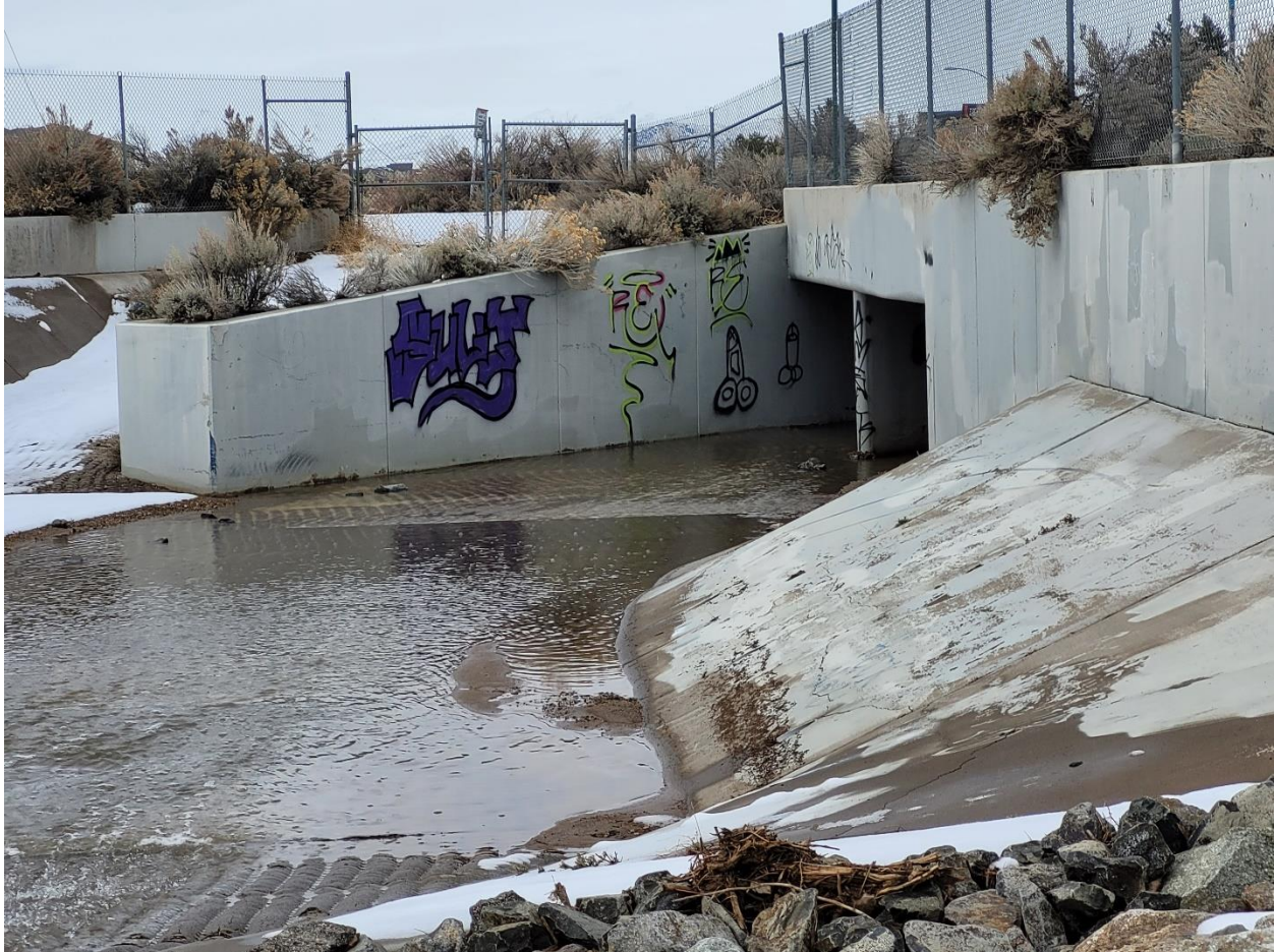
Inspection Site 8) Road crossing at Military Rd. is clean with no obstructions to impede water. (1/11/2023)
