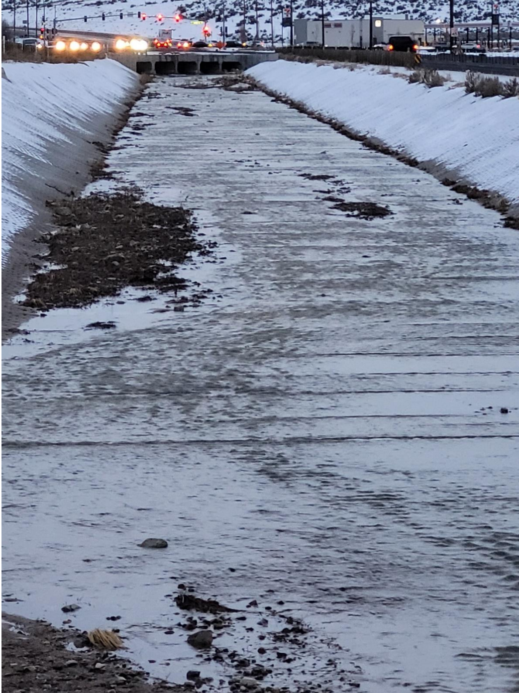
Inspection Site 2) Lemmon Valley drainage - picture of the road crossing under Lemmon Dr. near Lemmon Dr. and Military Rd. The channel is clear with no obstructions to impede water. (1/11/2023)
