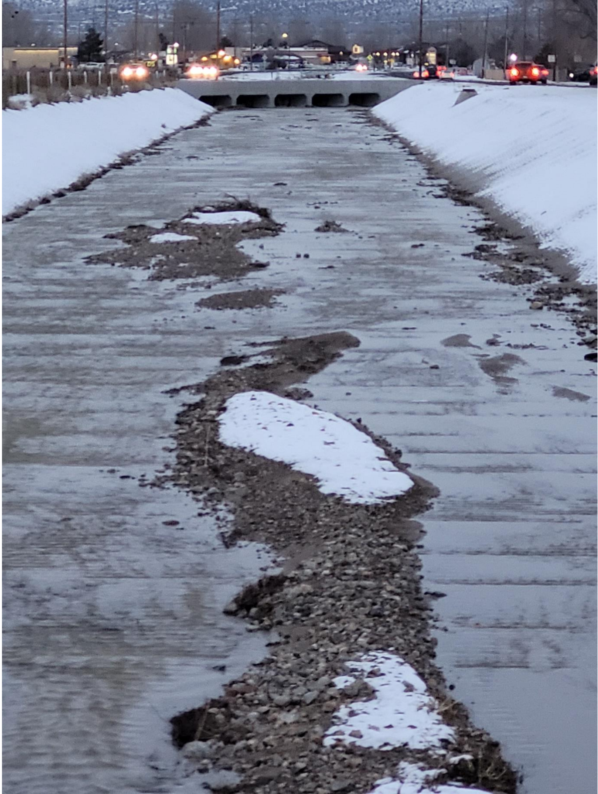
Inspection Site 3) Downstream road crossing under Lemmon Dr. heading north toward Swan Lake. The channel is clear with no obstructions to impede the water. (1/11/2023)
