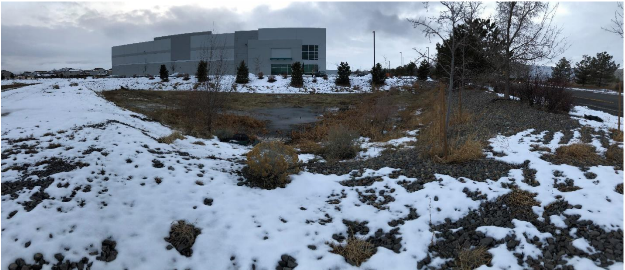
Inspection Site 11) Pictures taken on Monday 1/9/23 (top) and Wednesday 1/11/2023 (bottom) of the detention basin on the south side of Lear Blvd. This detention basin was nearly full on Monday, 1/9/23. The basin is functioning correctly, as it is almost empty in the picture taken on the following Wednesday inspection. (1/11/2023)
