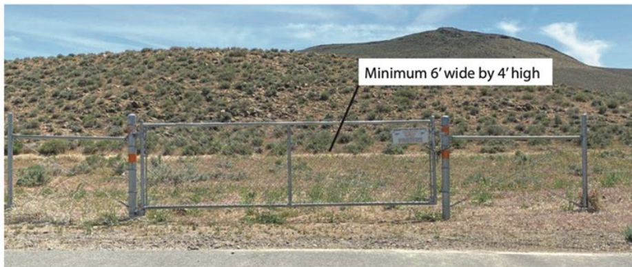
DETAIL C LOCKED EMERGENCY HORSE GATE
