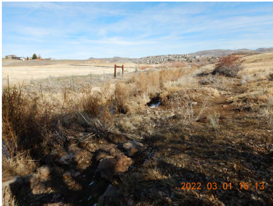
Photo 8. North Truckee Drain looking downstream at the pasture at the end of the project reach limits. Purple loosestrife ( Lythrum salicaria ) dominates the bank as observed from the property line.
