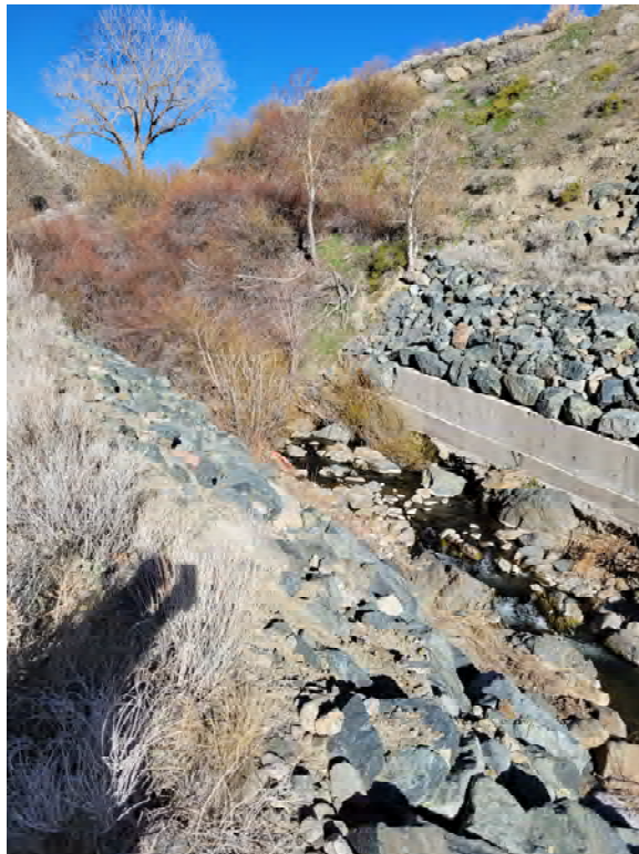
Photo 4. Looking upstream from outside the engineered channel.
