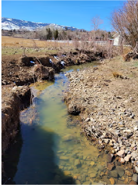
Photo 3. Looking upstream towards the adjacent private property. Willows stabilize the banks as South Evans Creek enters Anderson Regional Park.
