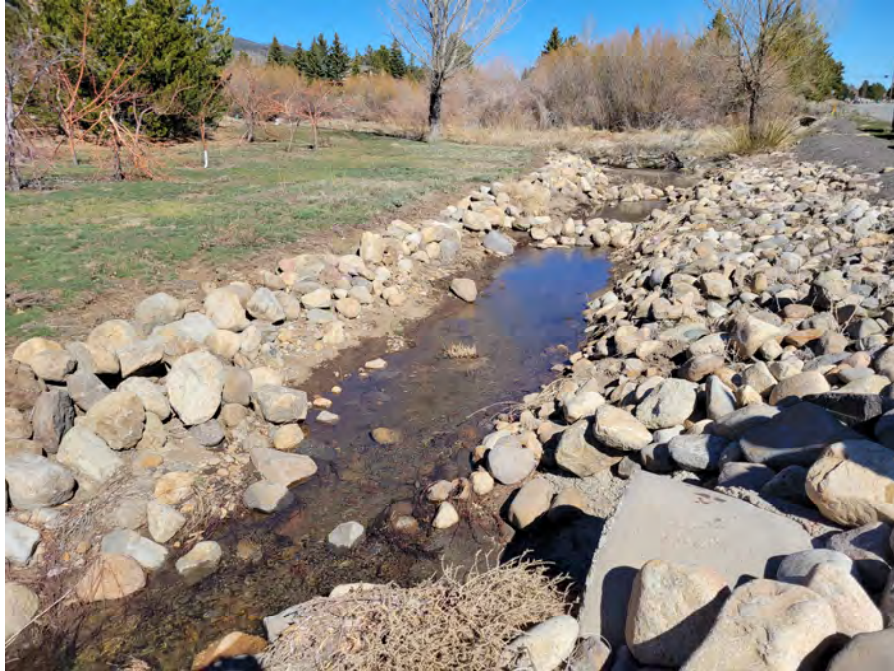
Photo 1. Upstream of Callahan Ranch Road, Jones Creek runs parallel to the road. The channel is lined with large cobble and check dams are present.
