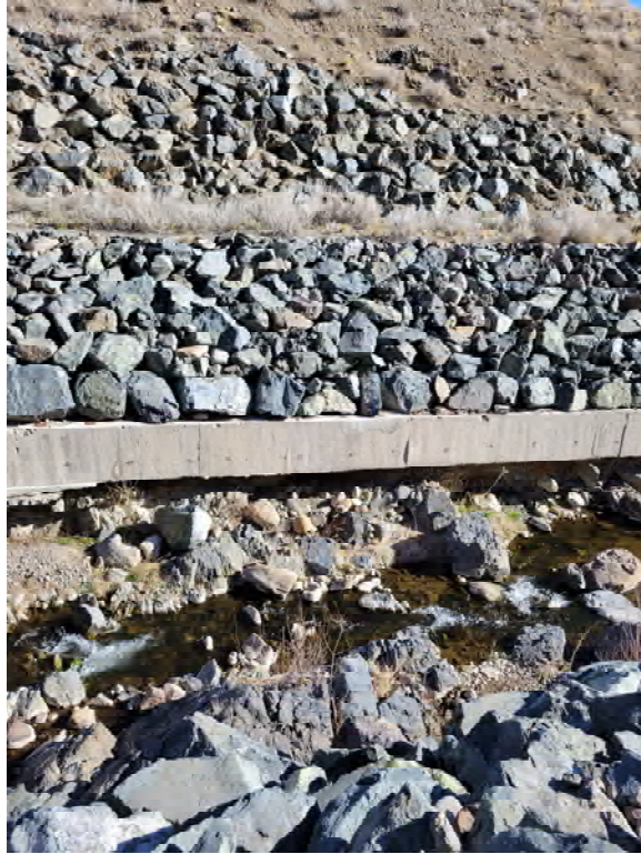
Photo 5. Looking north at the engineered channel.
