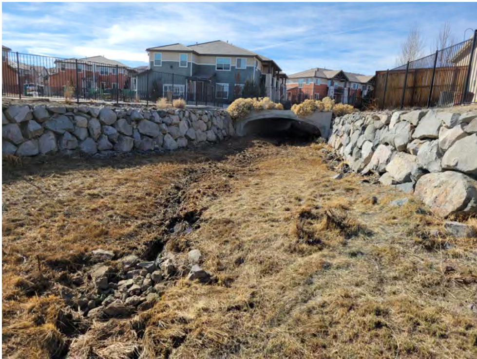
Photo 6. Drainage channel to the west of the North Truckee Drain was recently cleared. The area was documented to have purple loosestrife ( Lythrum salicaria ) and tall whitetop ( Lepidium latifolium ) in 2015.
