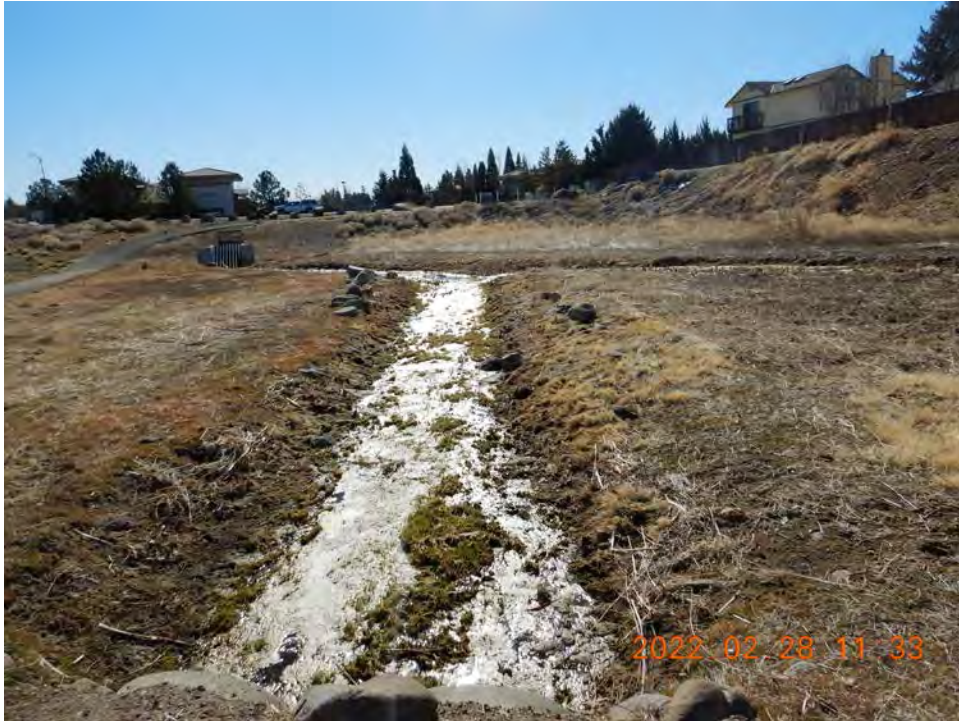
Photo 8. Chalk Creek looking downstream at Mae Anne Avenue outlet structure.
