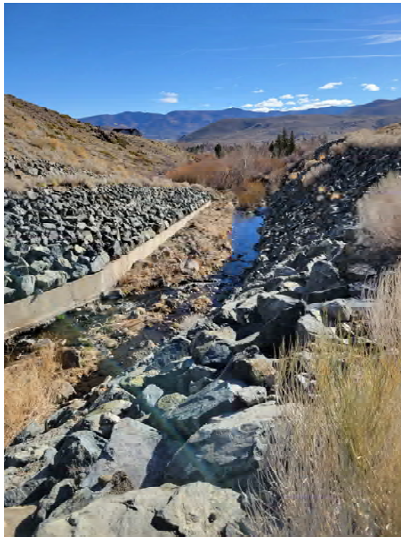
Photo 6. Looking downstream from outside the engineered channel.
