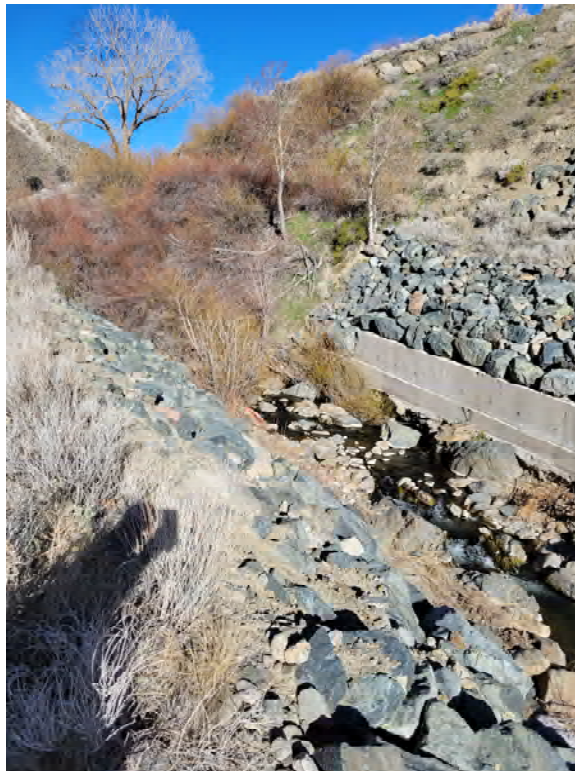
Photo 4. Looking upstream from outside the engineered channel.
