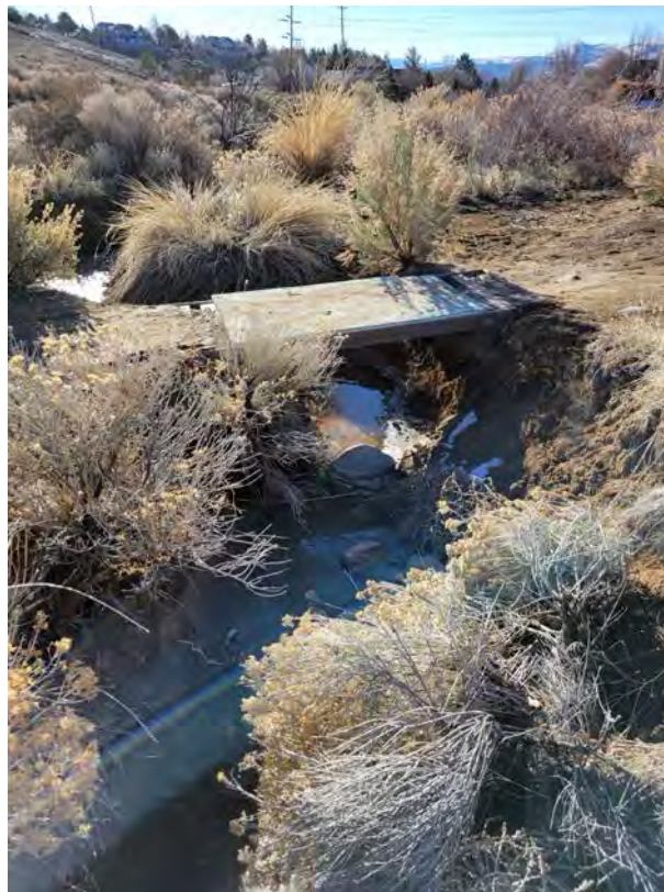
Photo 2. Western channel bypassing concrete grade control (Photo 1).
