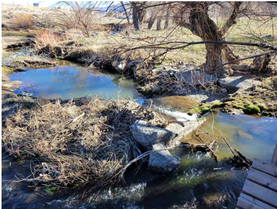
Photo 2. Existing weir downstream of the USGS gauge station. The majority of flow in Steamboat Creek bypasses the existing weir.
