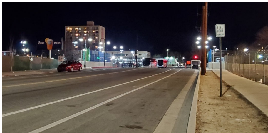
Exhibit 4. Ralston Street (looking north from Lot C exit)
