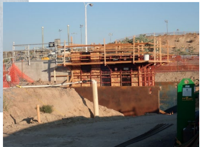
About Picture: Above - Looking NE & Down at launder rebar and forms placed at Secondary Clarifier #4 Right - Looking NW at forms installed for Splitter Box
