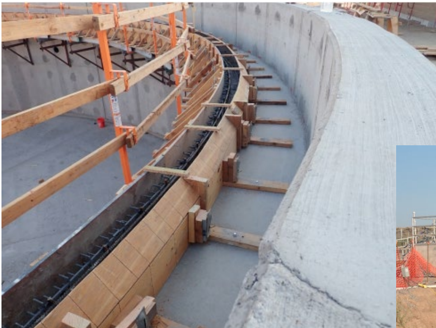
About Picture: Above - Looking NE & Down at launder rebar and forms placed at Secondary Clarifier #4 Right - Looking NW at forms installed for Splitter Box
