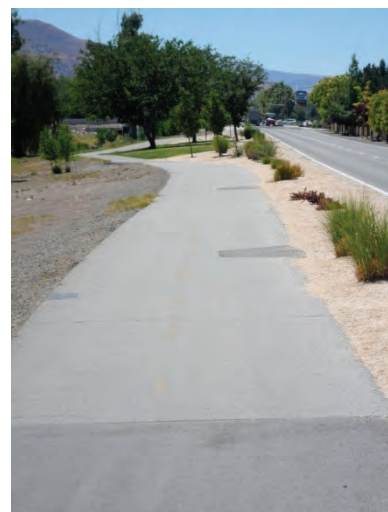
Shared-use Path Sparks Boulevard
