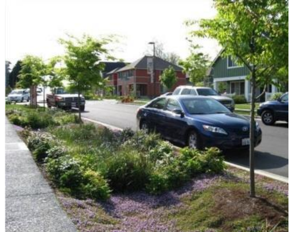
Vegetated swales along sidewalk. Source: Structural Controls and LID Manual (2015).
