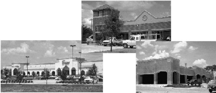
Figure 4-39: Building Façade Articulation
