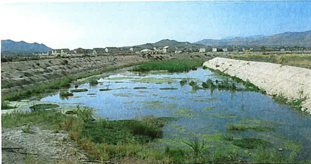
Photo 2. Sage Point Channel looking upstream from the end of Lear Blvd.
