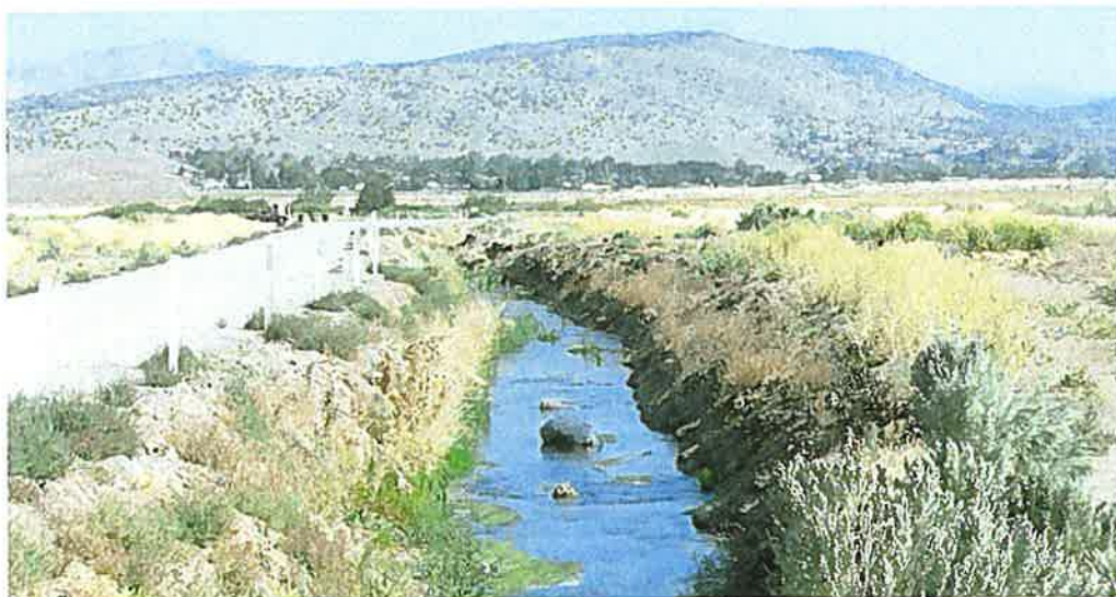
Photo 1. Horse Creek segment looking downstream from the end of Lear Blvd.
