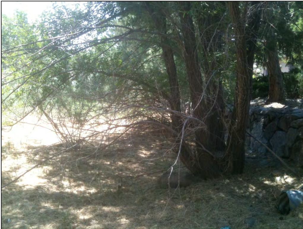
Looking upstream from Pheasant Lane culvert.
