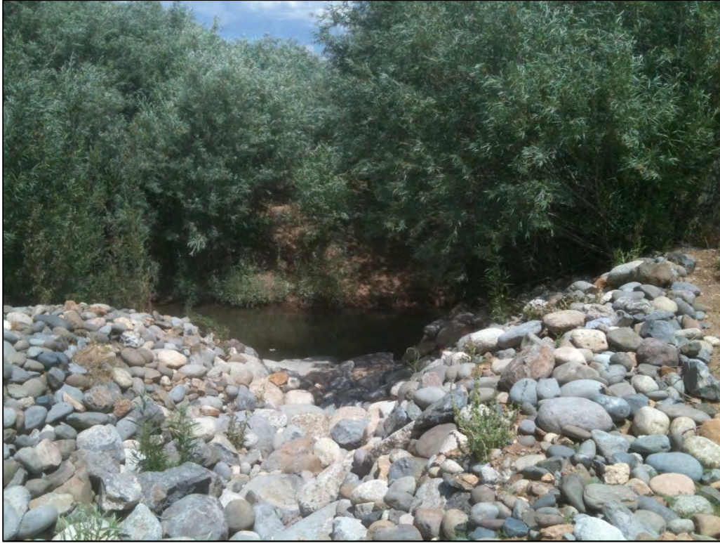
Dant Drainage connection to the Last Chance Ditch.
