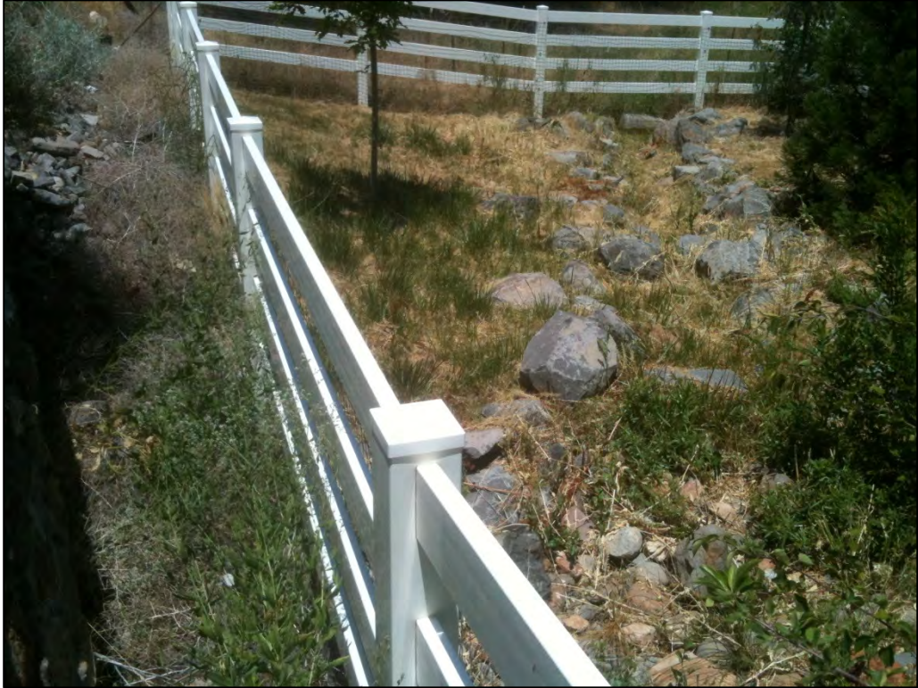
Ranch fence 2-3 ft downstream of Pheasant Lane culvert.
