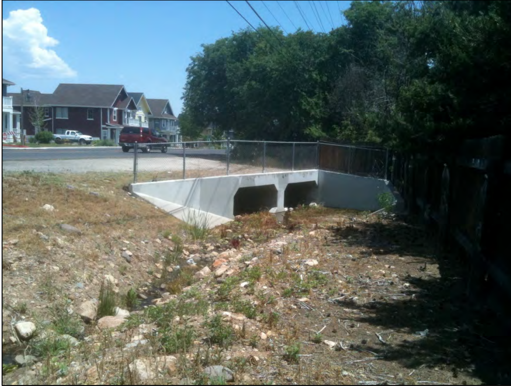
West Moana Lane culverts.
