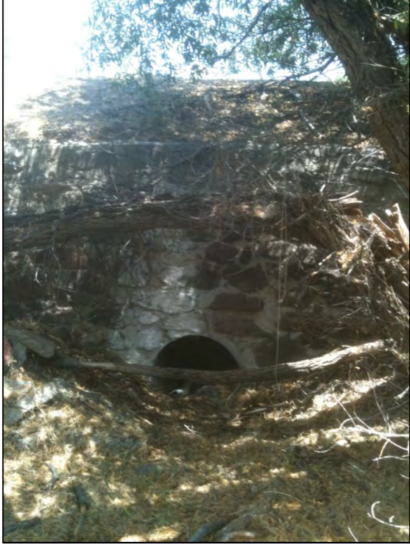
Upstream Headwall of Pheasant Lane 27" CMP culvert.
