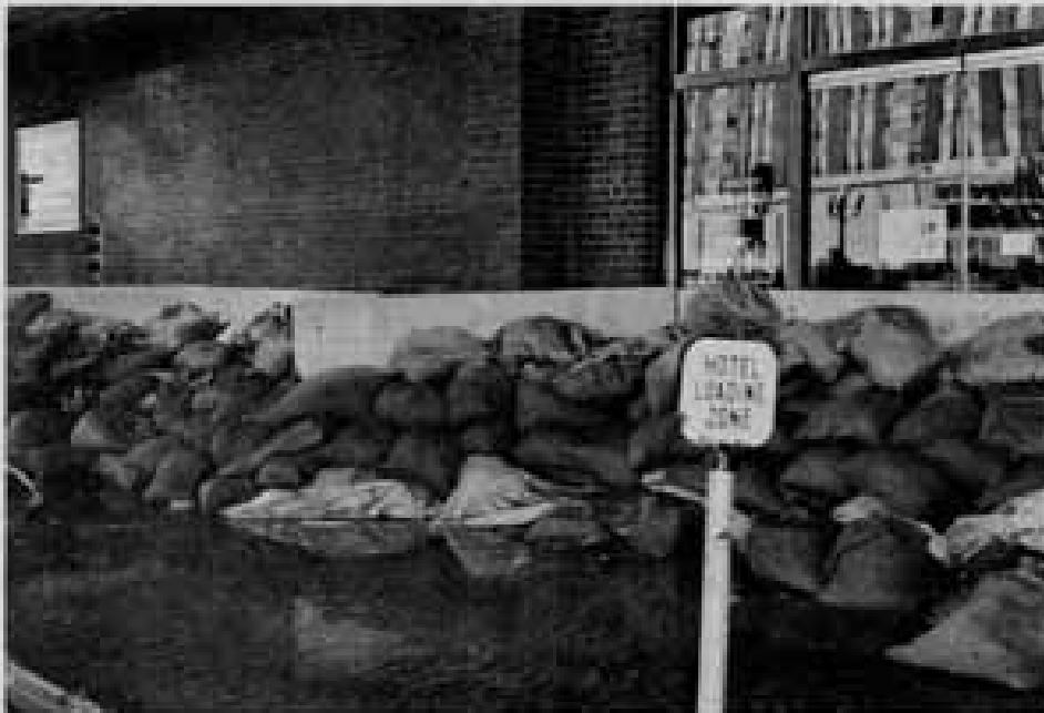
Figure 15. Sandbag barrier emplaced to protect the Riverside Hotel during the February 1963 flood. (Reno Evening Gazette photo)
