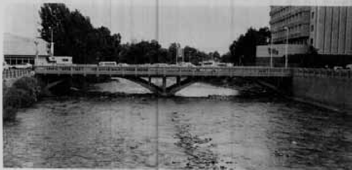
Figure 22. Center Street Bridge.
