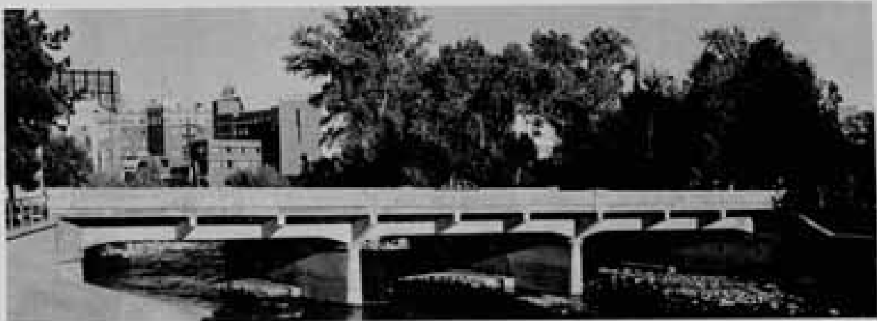
Figure 19. Arlington Avenue Bridge.
