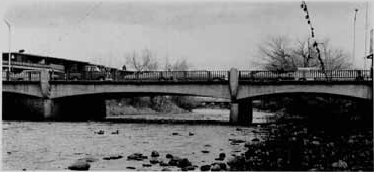
Figure 23. Lake Street Bridge showing removable handrails.
