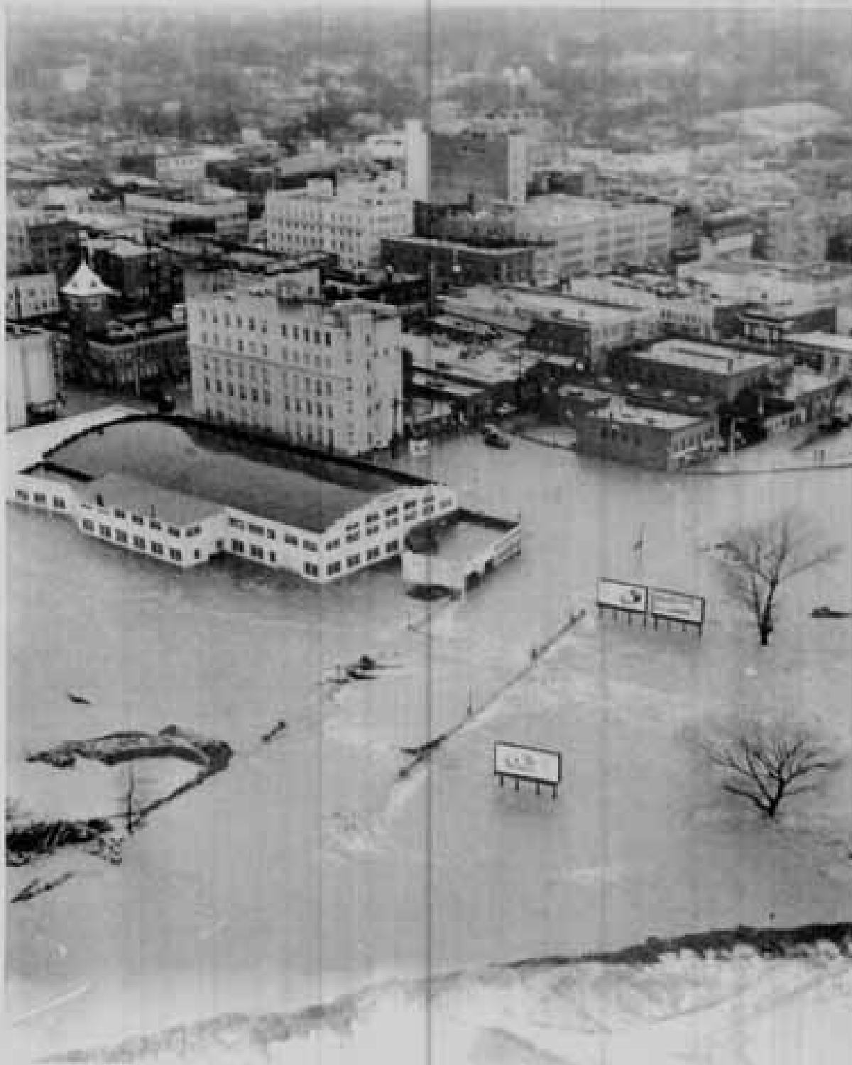
Figure 13. Flooding in the vicinity of the Lake Street Bridge, December 1955. (Photo courtesy of the Silver State Press)
