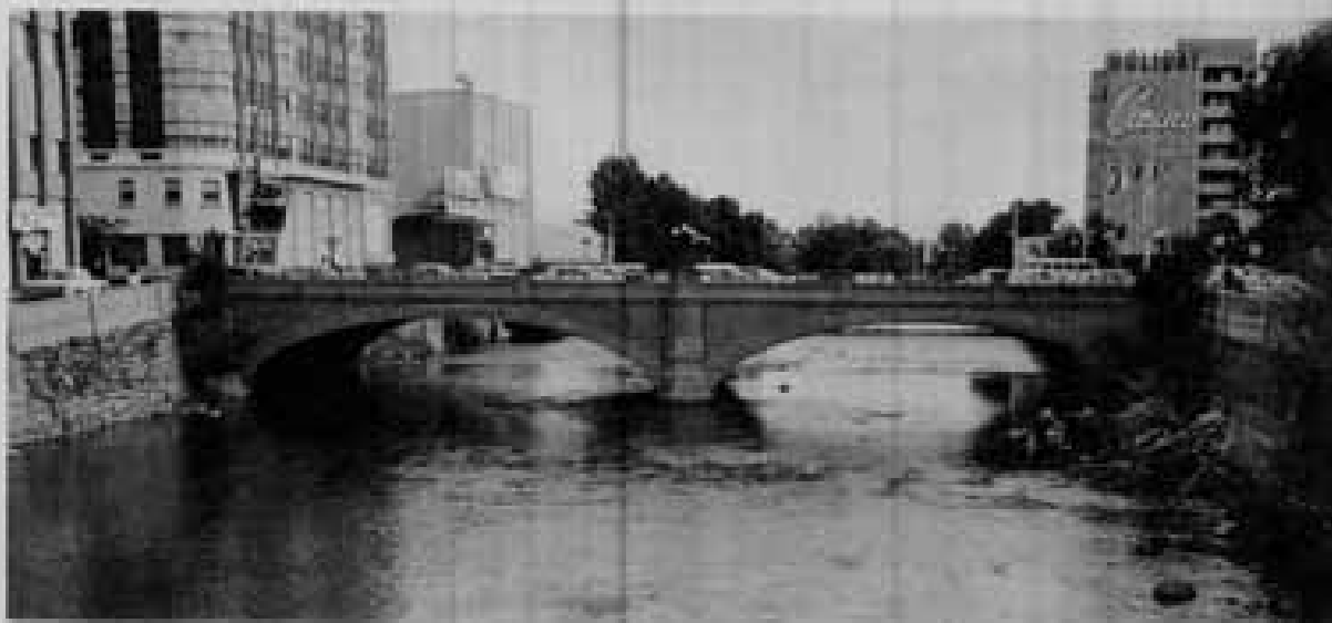
Figure 21. Virginia Street Bridge.
