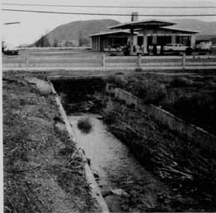
Figure 29. Culvert on Evans Creek at South Virginia Street.
