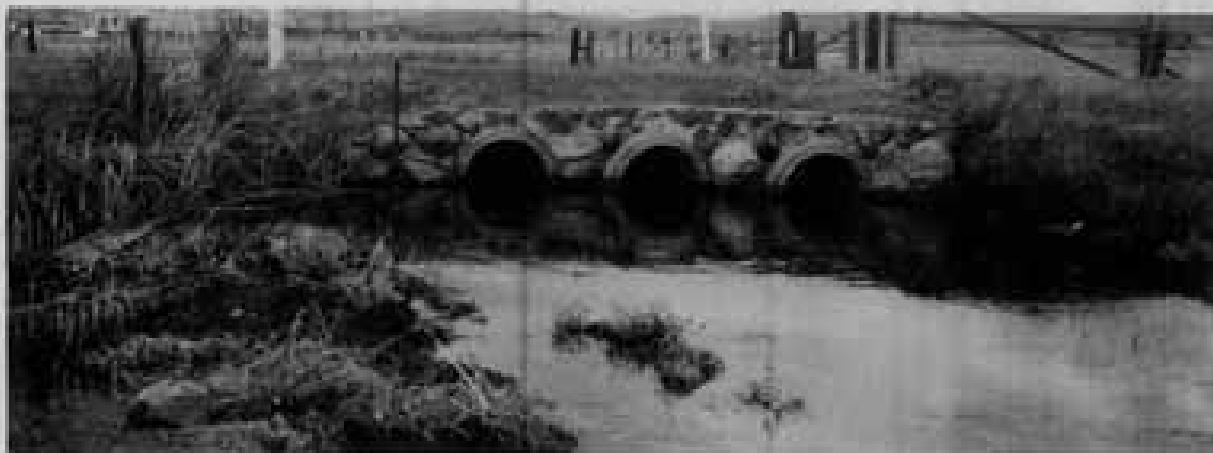
Figure 31. Culvert on North Truckee Drain at Prafer Way.
