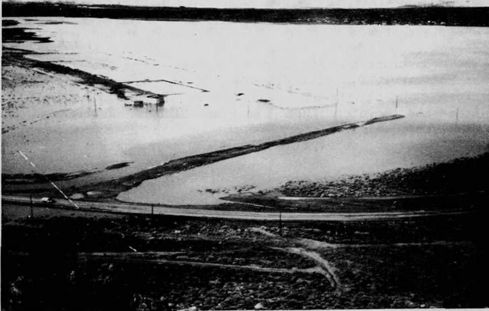
Figure 20. Flooding of sewage treatment plant in Lemmon Valley Playa. February 1986. (Photo by Nimbus Engineers)
