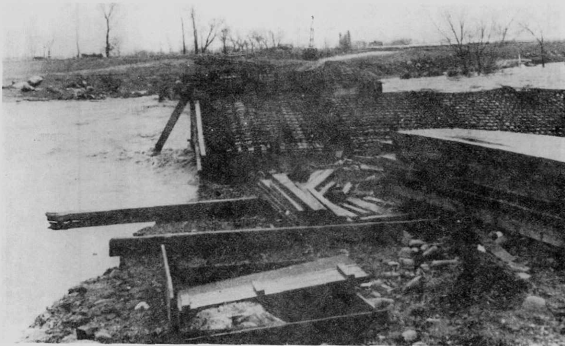
Figure 13. One of the major losses of the December 1955 flood was the newly completed Kietzke Lane Bridge.
