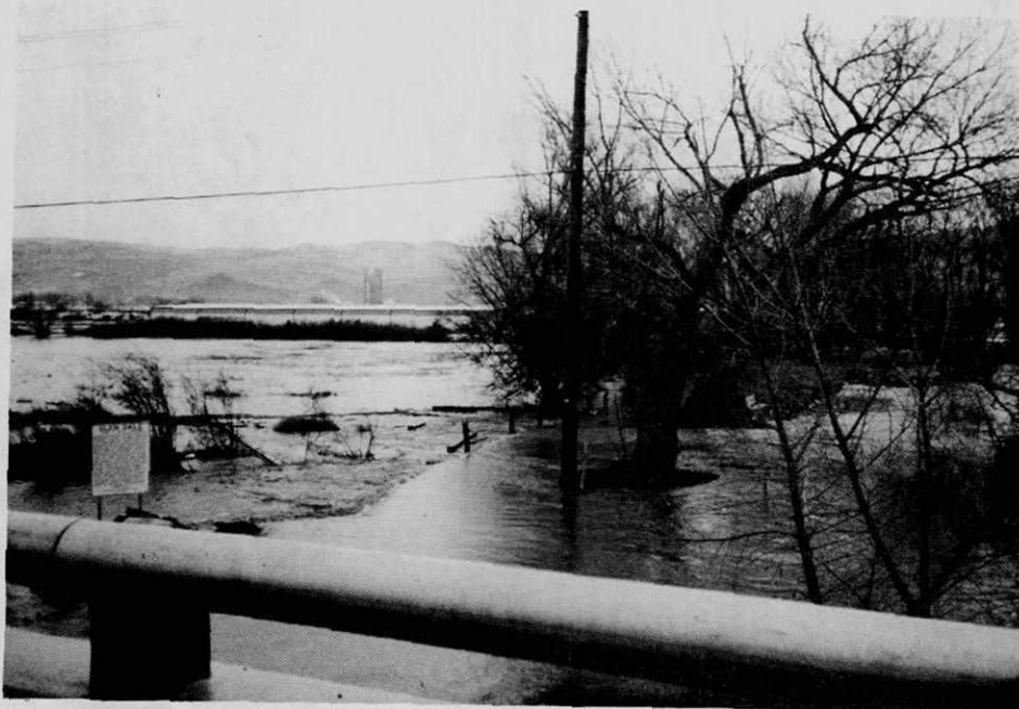
Figure 18. Overflow from the Truckee River. Downstream of McCurran Boulevard Bridge, February 1986. (Photo by Nimbus Engineers.)
