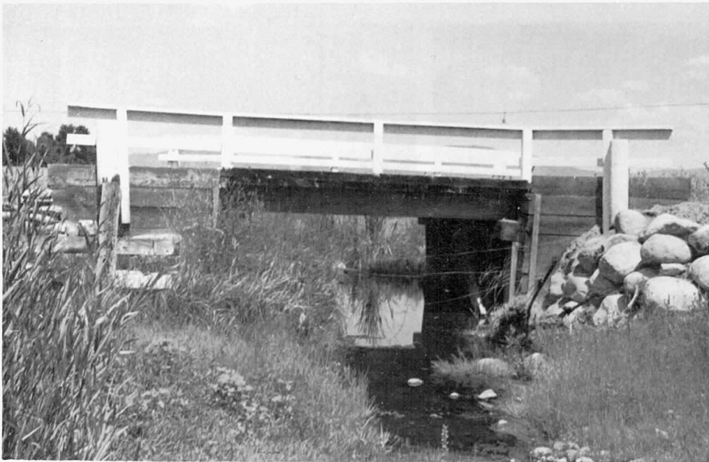
Figure 3 - Bridge over Dry Creek at Timothy Lane.
