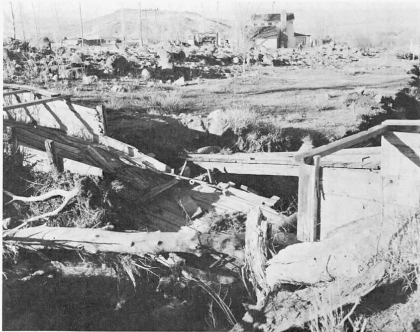
Figure 7 - Remains of Steamboat Ditch Flume crossing of Thomas Creek following the January-February 1963 floods. Rock debris from earlier cloudburst floods appears in the background (Soil Conservation Service photo).
