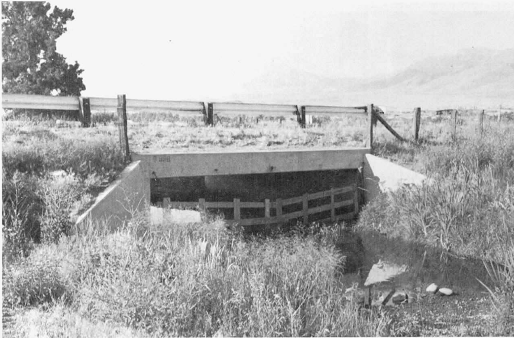
Figure 2 - Culvert on Dry Creek at Huffaker Lane.
