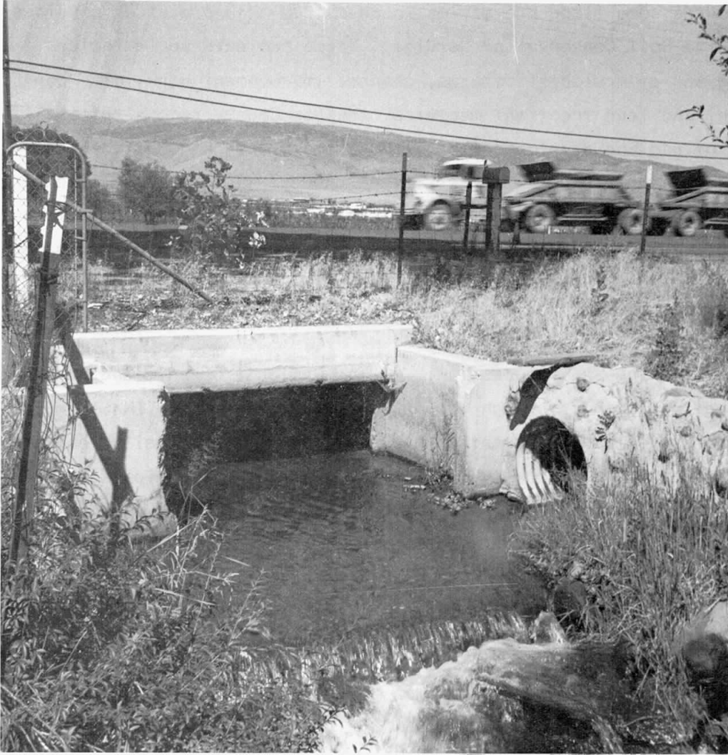
Figure 6 - Culvert on Whites Creek at Highway 395.
