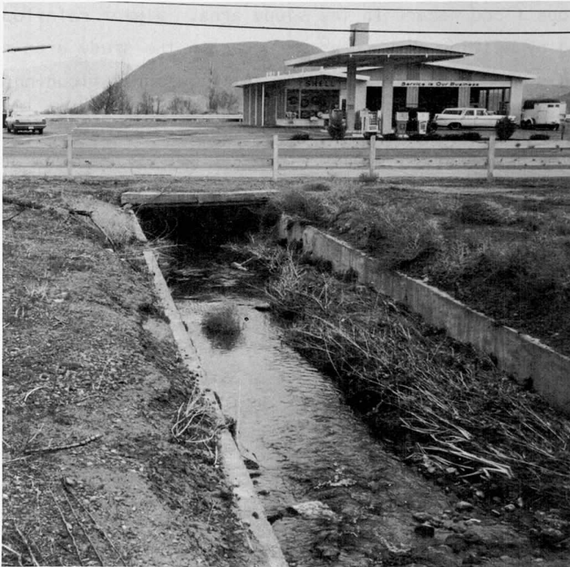
Figure 1 - Culvert on Evans Creek at Highway 395.
