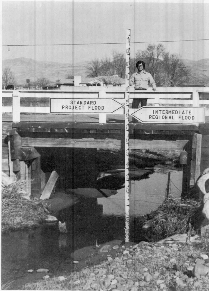
Figure 11 - Future flood heights, Dry Creek at Timothy Lane.
