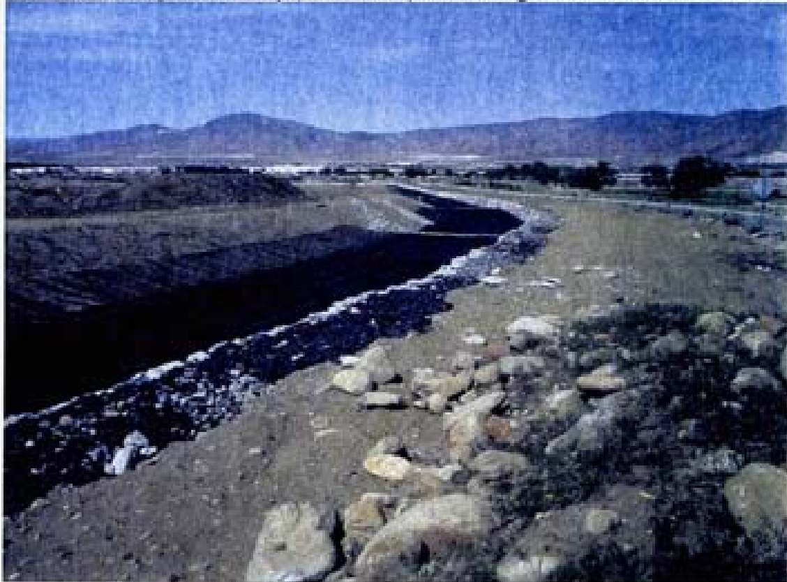
Figure 2. Looking northeasterly (downstream) of the realigned Whites Creek Branch 2
