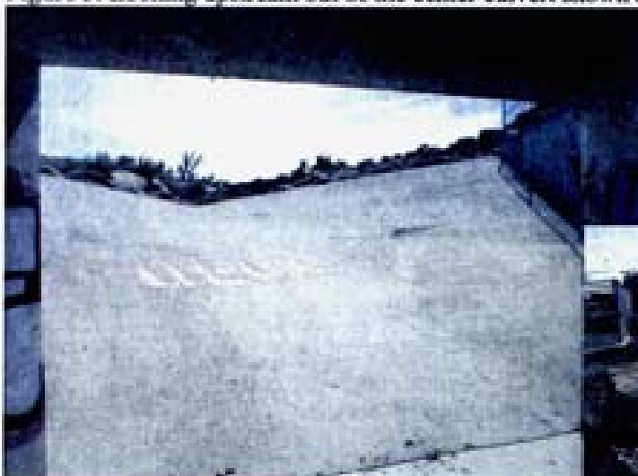
Figure 5. Looking upstream out of the center culvert shown above.
