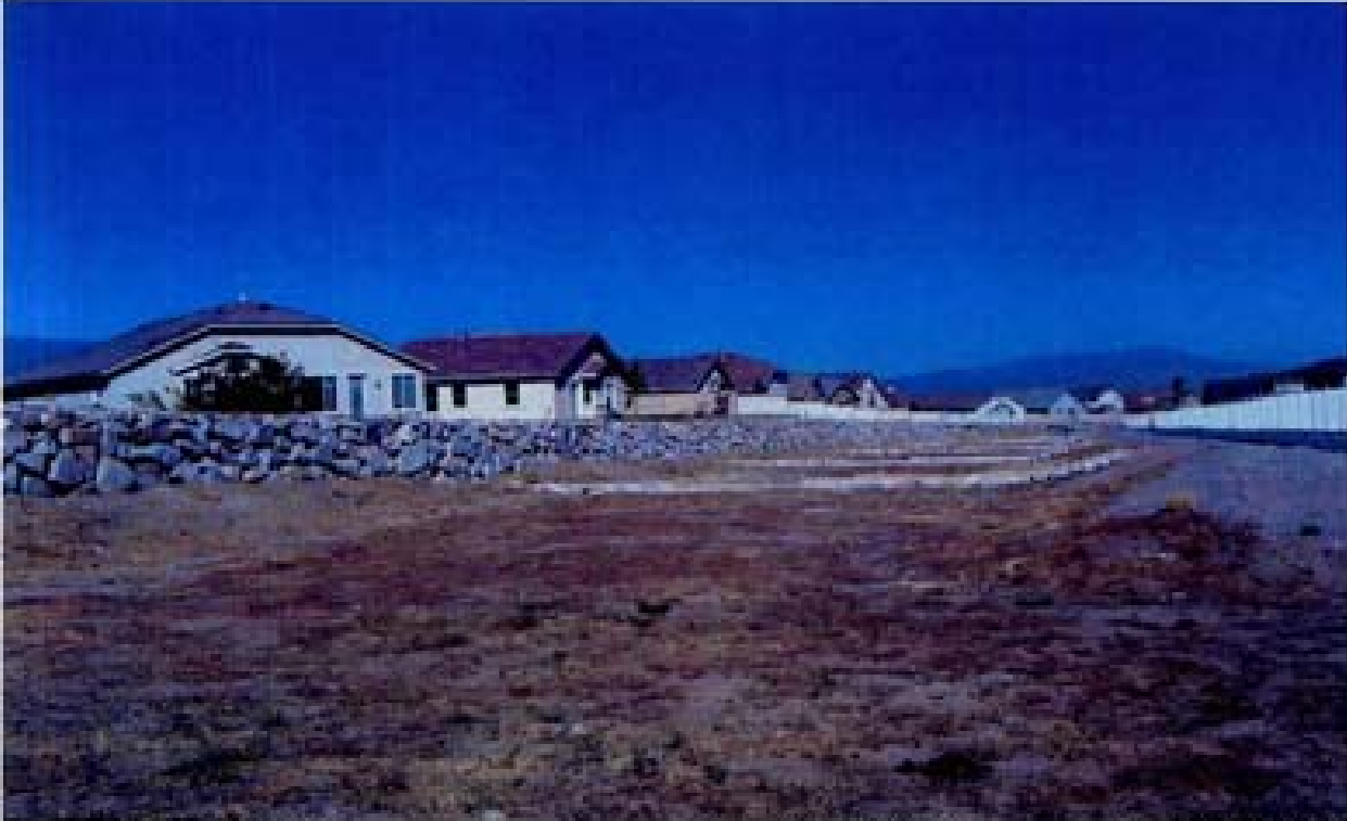
Title: Site 11 - Channel SE-8A File: HPIM2257.JPG Date: 8/22/2008 10:15 Desc: Slide: 2256 Facing Northerly; facing down gradient. Rockery wall encroaches into channel for the entire length.
