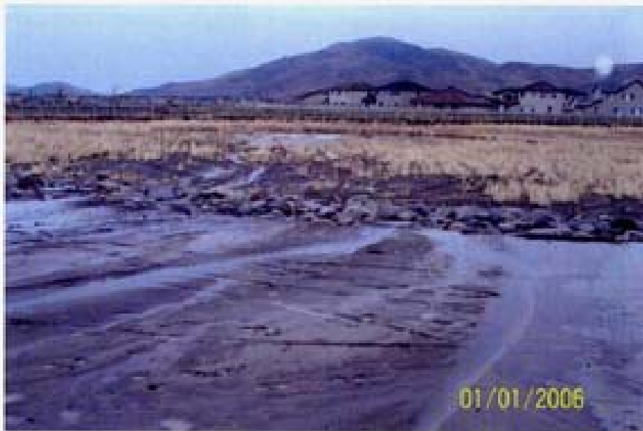
Photo 63. 1/1/06 - Close up of sediment discharge to wetland DE 4 after 12/31/05 storm event.
