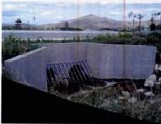
Culvert entrance under Rio Wrangler
