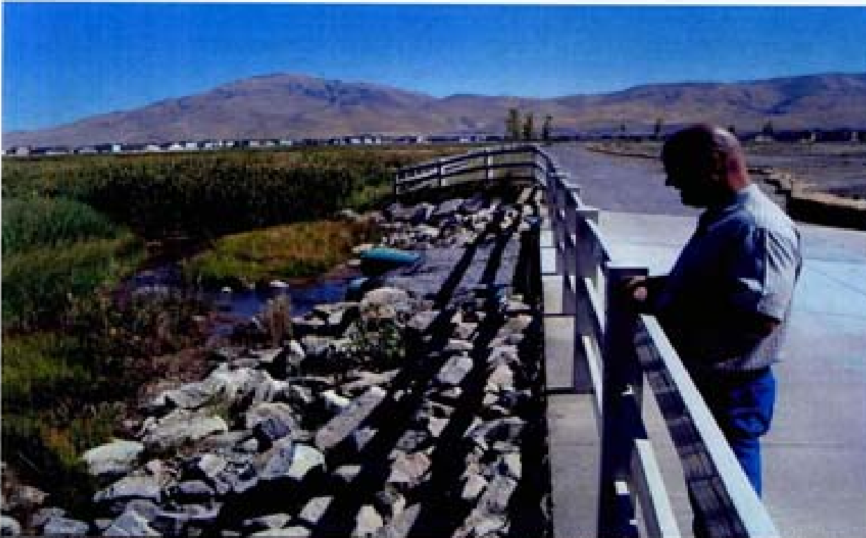
Title: Site 8 - Channel W1-B File: HPIM0260.JPG Date: 8/22/2006 10:54 Desc: Slide: 2267 Facing Easterly; end of channel W1-B. Newly constructed low flow PVC culverts under sawcut portion of pedestrian path.
