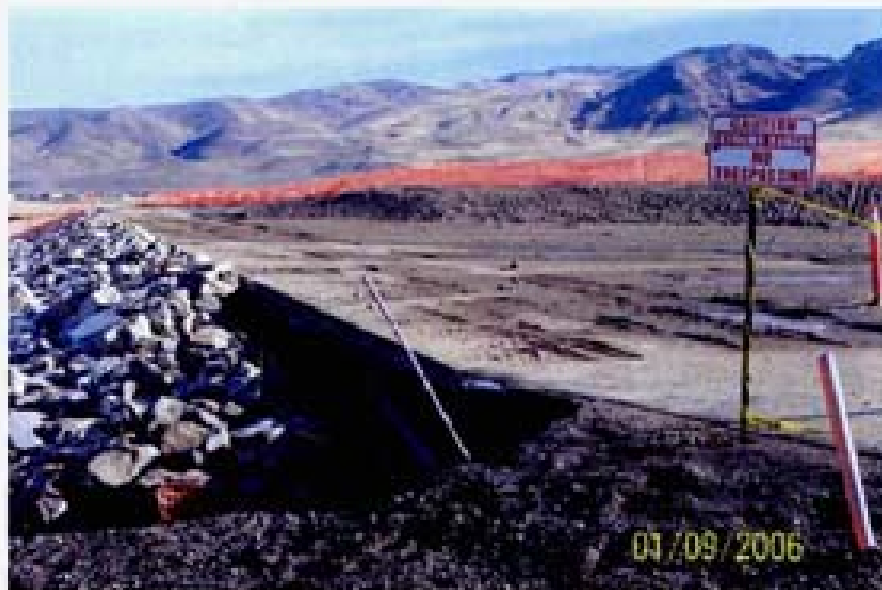
Photo 88, 1/9/06 - Erosion of the channel C-7 drop structure after the 12/31/05 storm event. Note the light purple recycled water line is exposed. View looking east.
