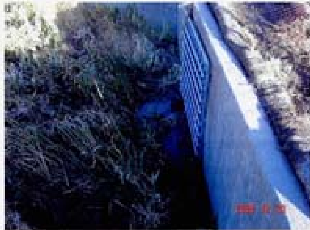
Culvert headwall in Dec. 2005
