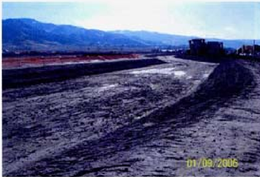
Photo 91, 1/9/06 - The lower end of unprotected channel C-7 after the 12/31/05 storm event. View looking southeast.
