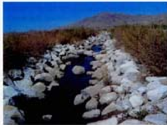
The middle stretch of the W1-B channel
