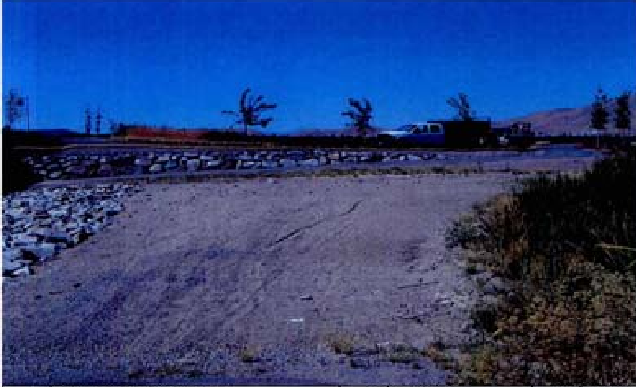
Title Site 3 - Detention basin RCB culvert outlet File HPM2204.JPG Date 8/15/2006 15:54 Desc: Slide 2204 Facing northerly, portion of pedestrian/bike path.
