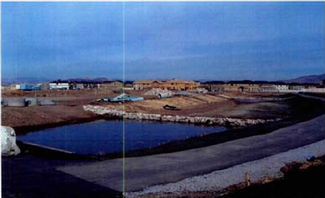
Title: Site 7 Channel C-5 File: HPM02582.JPG Date: 11/12/2006 10:59 Desc: Slide: 2582 Facing Northerly; outlet from RCB into beginning of C-5 Channel. Grade control sill has been constructed improperly and grading of channel is questionable and is causing water to be blocked/ponded by grade control sill.
