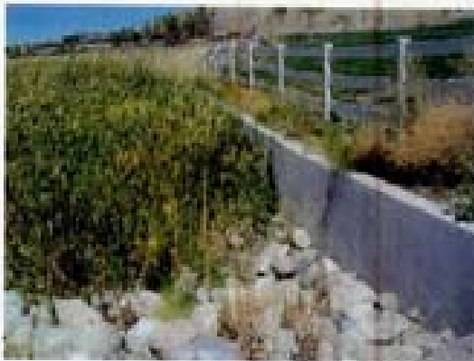
Outlet of twin RCB's August of 2005
