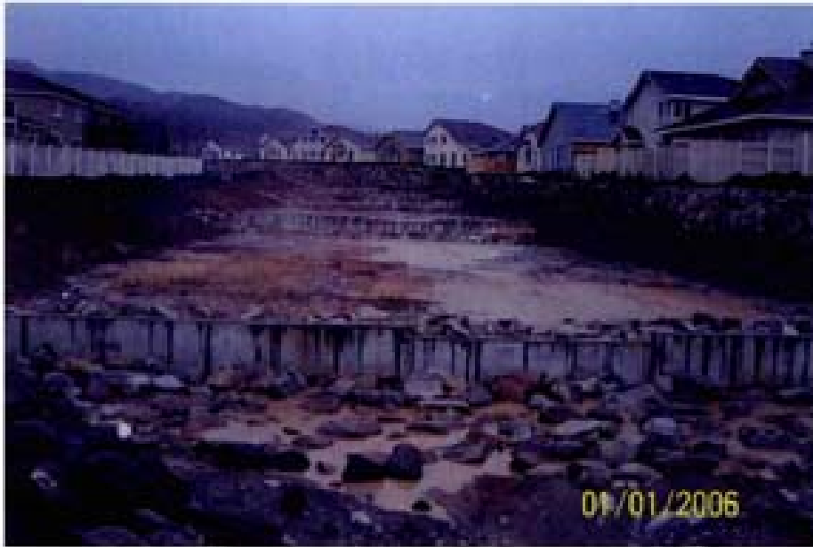
Photo 54. 1/1/06 - Low grade control structures on channel SE 8A above Rio Wraugler Parkway after 12/01/05 storm event. View looking south.
