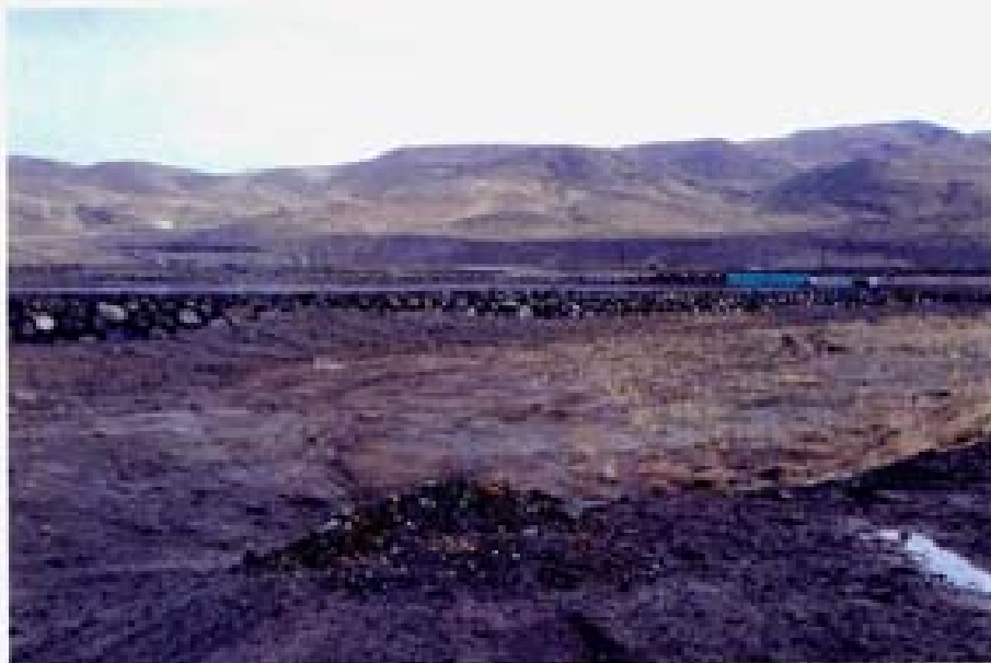
Photo 27. 12/5/05 - Flood control channel above Rio Wrangler Parkway with new construction in the background. View looking northeast.
