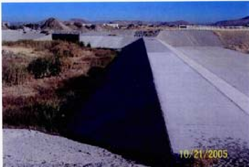
Photo 1. 10/21/05 - Overflow weir and culvert structure on Streamboat Creek at upper west end of detention basin. View looking north.
