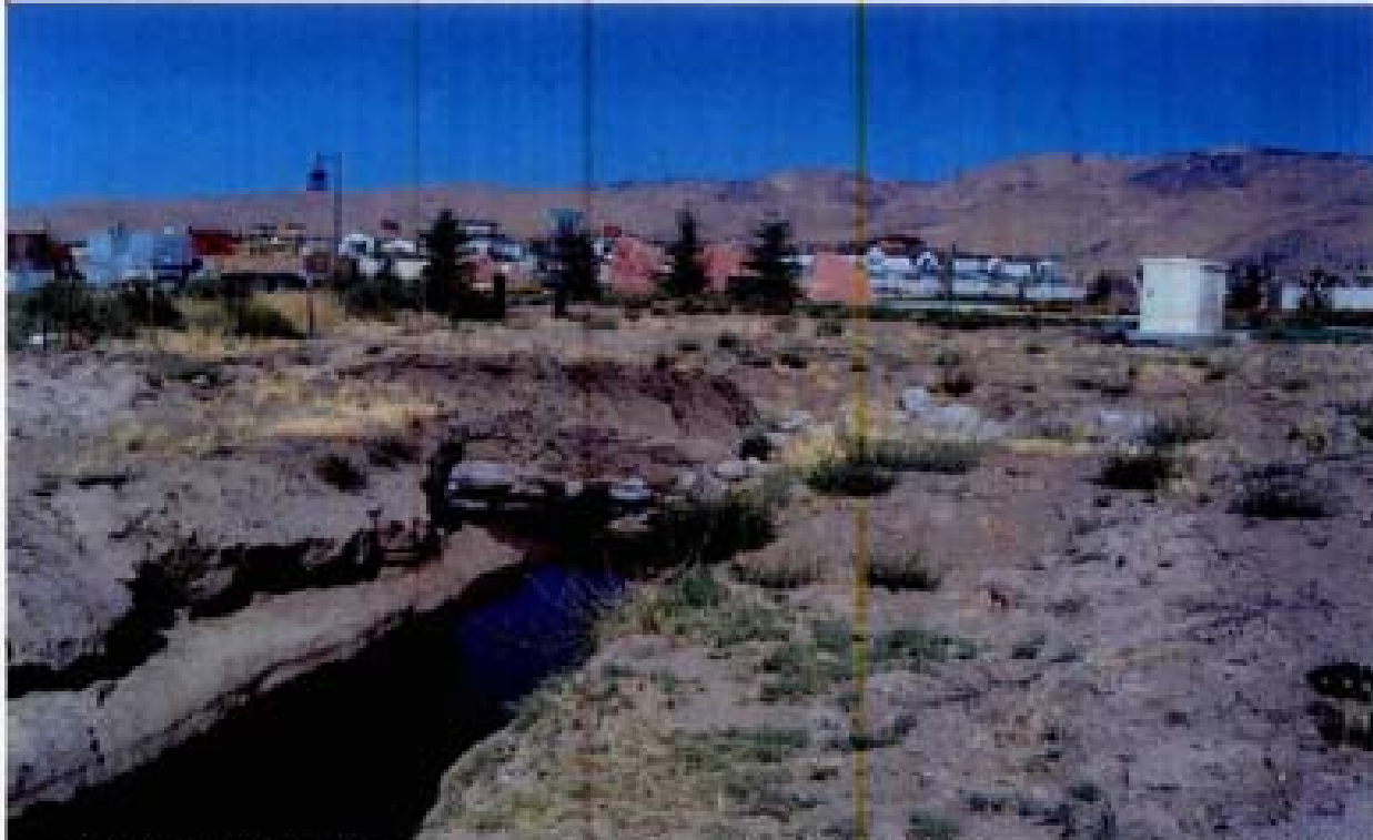
Title: Site 5 - Crane & Clow Ditch File: HPIM2214.JPG Date: 8/15/2008 16:15 Desc: Slide: 2214 Facing Easterly; same location as Photo 2213. This is the portion of ditch constructed as part of the development to supply water to D65. This ditch shows signs of being very unstable. Highly erodible layer of soil ~3 feet thick overlays a more stable, cohesive layer underneath as seen in left of photo.
