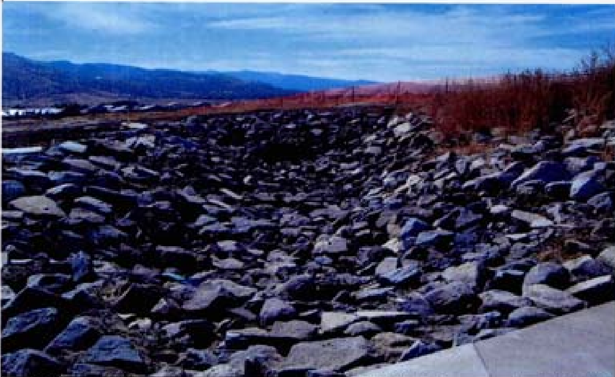
Title: Site 8 - Channel W1-B File: HPIM0270.JPG Date: 8/22/2006 10:55 Desc: Slide: 2268 Facing SEasterly; portion of channel W1-B just up gradient of pedestrian path. Temporary crossing with steel pipe visible in center of photo.
