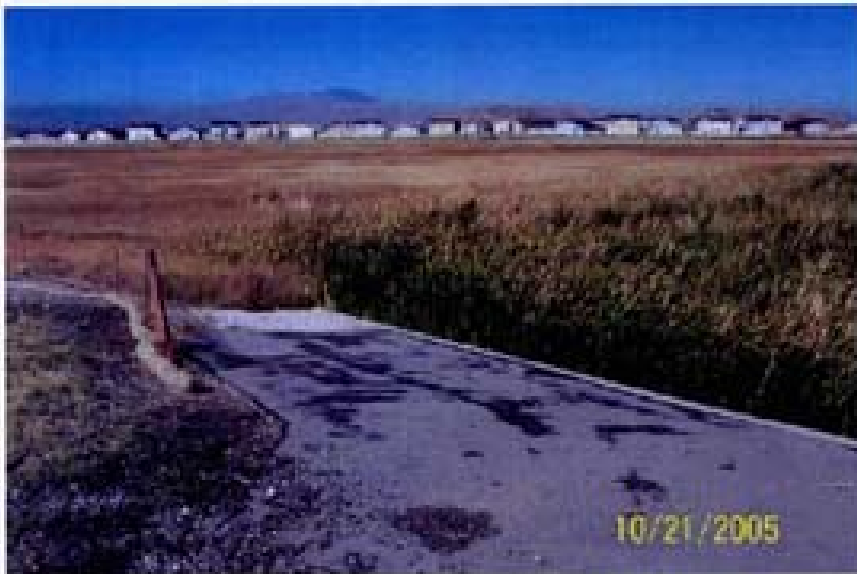
Photo 48, 10/21/05 - Paved maintenance access next to culvert outlet on south side of wetland DE3. View looking north.
