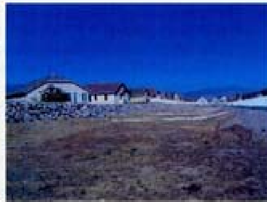
Looking downstream from intersection with south boundary channel
