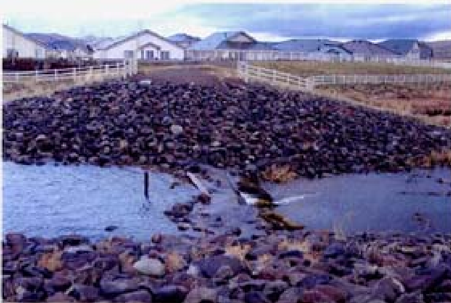
Photo 45. 12/1/05 - Web between wetlands DE1 and DE3. View looking north.
