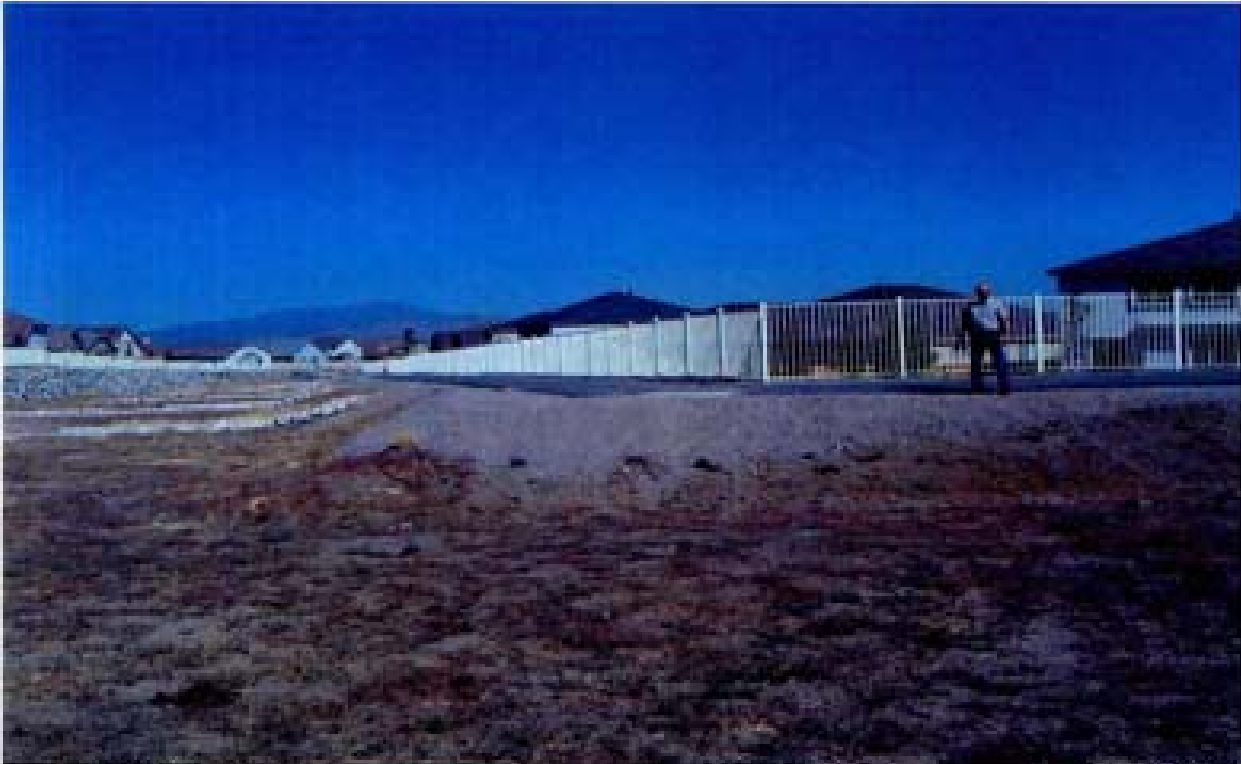
Title: Site 11 - Channel SE-8A File: HPIM2256.JPG Date: 8/22/2008 10:15 Desc: Slide: 2255 Facing Northerly; intersection of channel SE-8A and South boundary collection channel. Pedestrian path too sharp for a vic truck to make the turn. Vegetation is sparse to moderate density.
