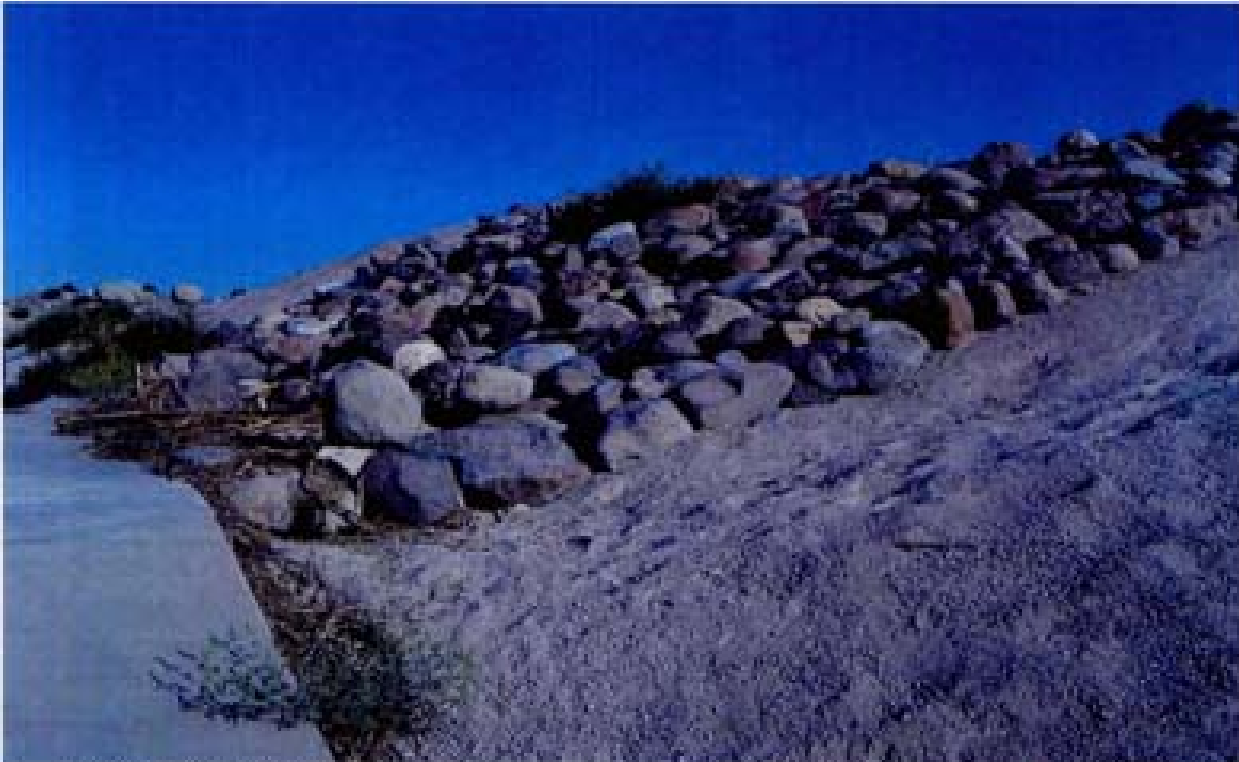
Title Site 1 - Diversion Structure File HPM02235.JPG Date 8/22/2008 8:40 Desc: Facing NWesterly; rock on slope at North end of diversion structure.
