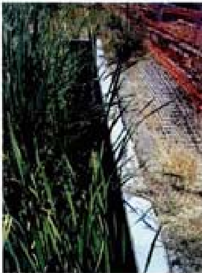
Culvert outlet in Sept. 2006
