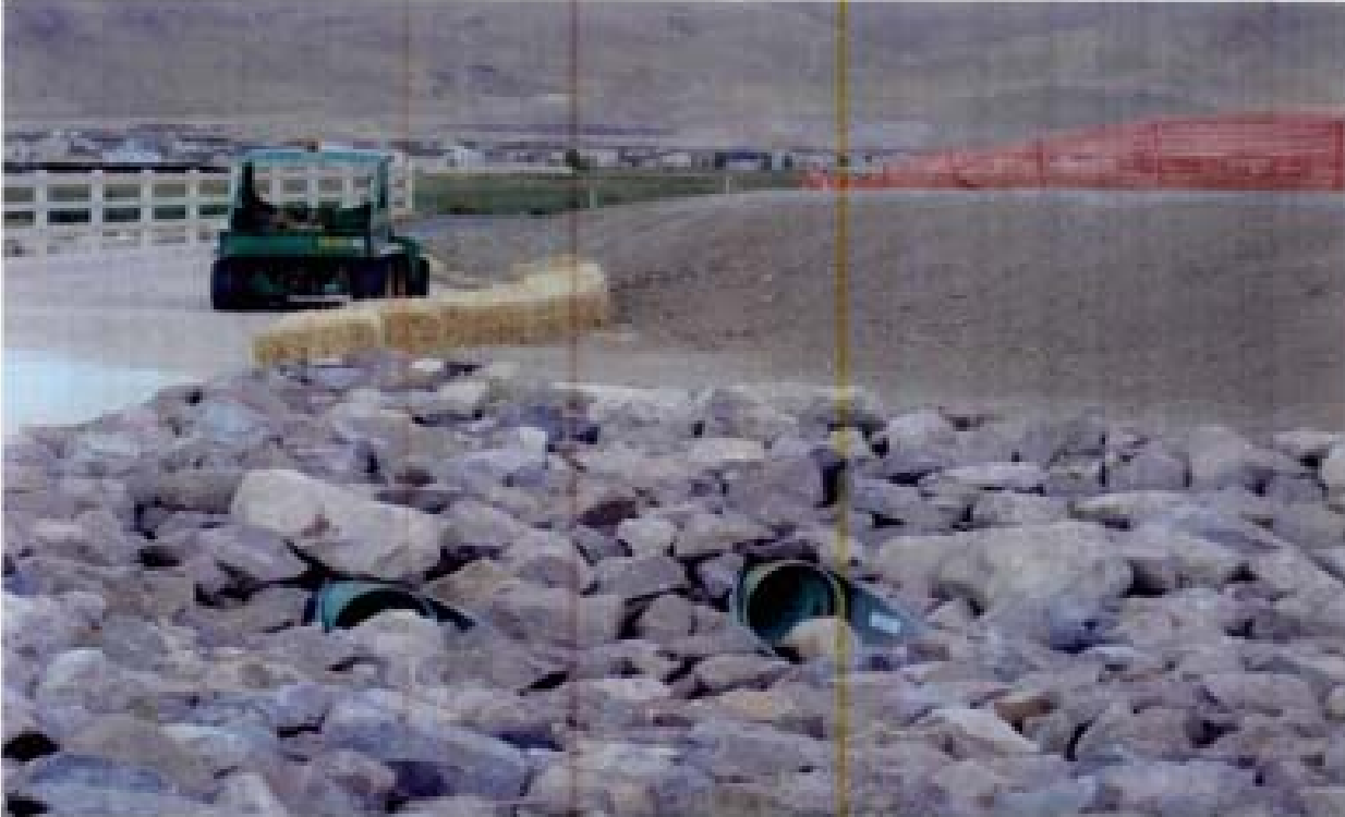
Title: Site 8 - Channel C-7 File: P1010174.JPG Date: 9/15/2006 15:17 Desc: Slide: 1010174 Same as Photo 1010174. Close up of PVC culvert inlets.
