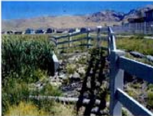
Culvert headwall at DE4 wetland
