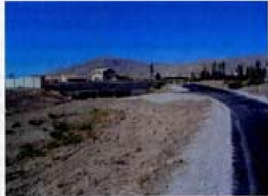
End of C-5 channel at Rio Wrangler
