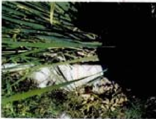
Top of headwall
