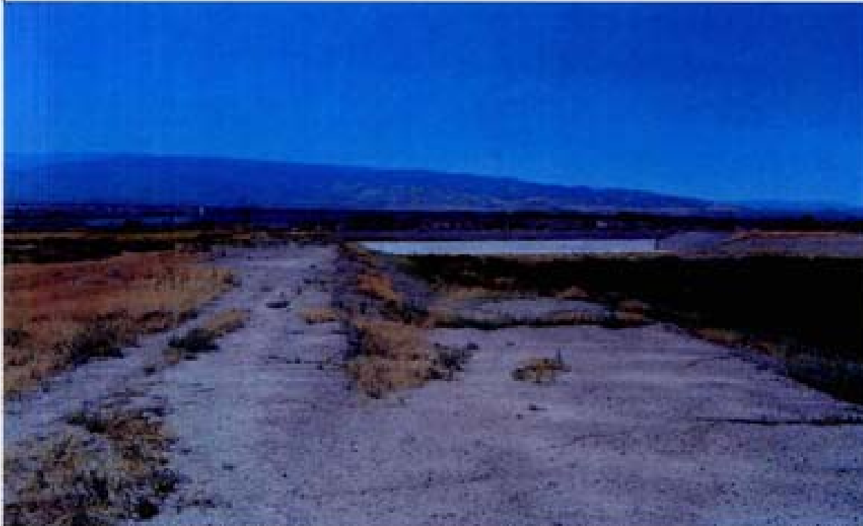
Title: Site 1 - Detention basin diversion structure File: HPIM2188.JPG Date: 8/15/2008 15:22 Desc: Slide: 2188 Facing Westerly; Access road into bottom of basin. Access road is not stabilized. Sparse vegetation on slope adjacent to the basin access road.
