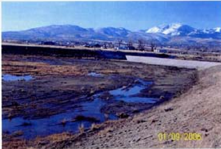
Photo 4, 1/9/06 - Upper west end of detention basin after 12/31/05 storm event where flows spilled over weir. View looking southwest.
