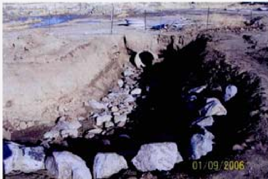
Photo 70, 1/9/06 - Diversion in Crane & Crow ditch 90' from previous photo. View looking north.
