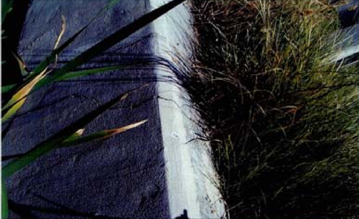
Title: Site 18 - RCB outlet across from Damonite High School File: HPM02290.JPG Date: 8/22/2008 13:37 Desc: Slide: 2288 Facing Northerly; front face of the headwall/wingwall intersection. Large crack at the section where the headwall is formed with the wingwall. This crack is large (can fit a nickel) and appears to go through the thickness of the wingwall.
