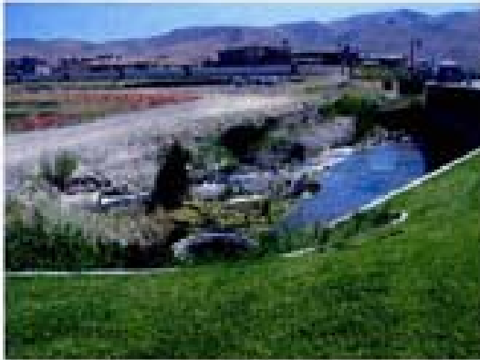
RCB outlet under Steamboat Parkway
