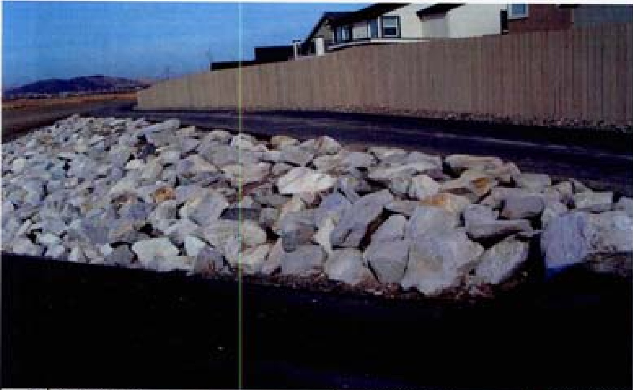
Title: Site 10 W-3 Channel File: HPM2598.JPG Date: 11/13/2006 11:12 Desc: Facing Northerly; from the access ramp pictured above. Riprap on slope downstream of the access ramp.
