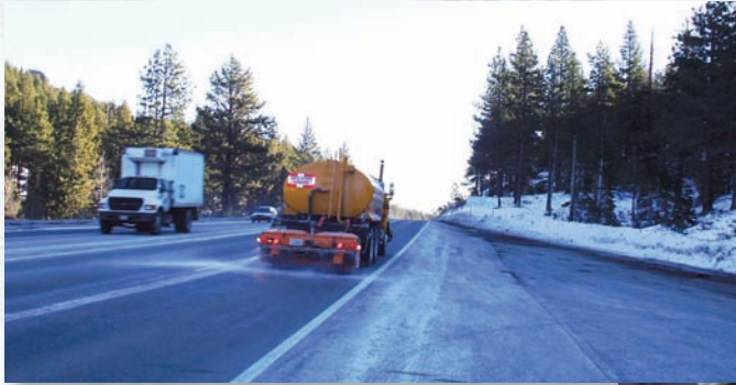
A Nevada Department of Transportation truck applies liquid brine solution to the highway in anticipation of another snow storm.
