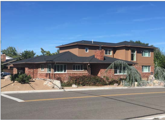
Example: Renovations and additions
